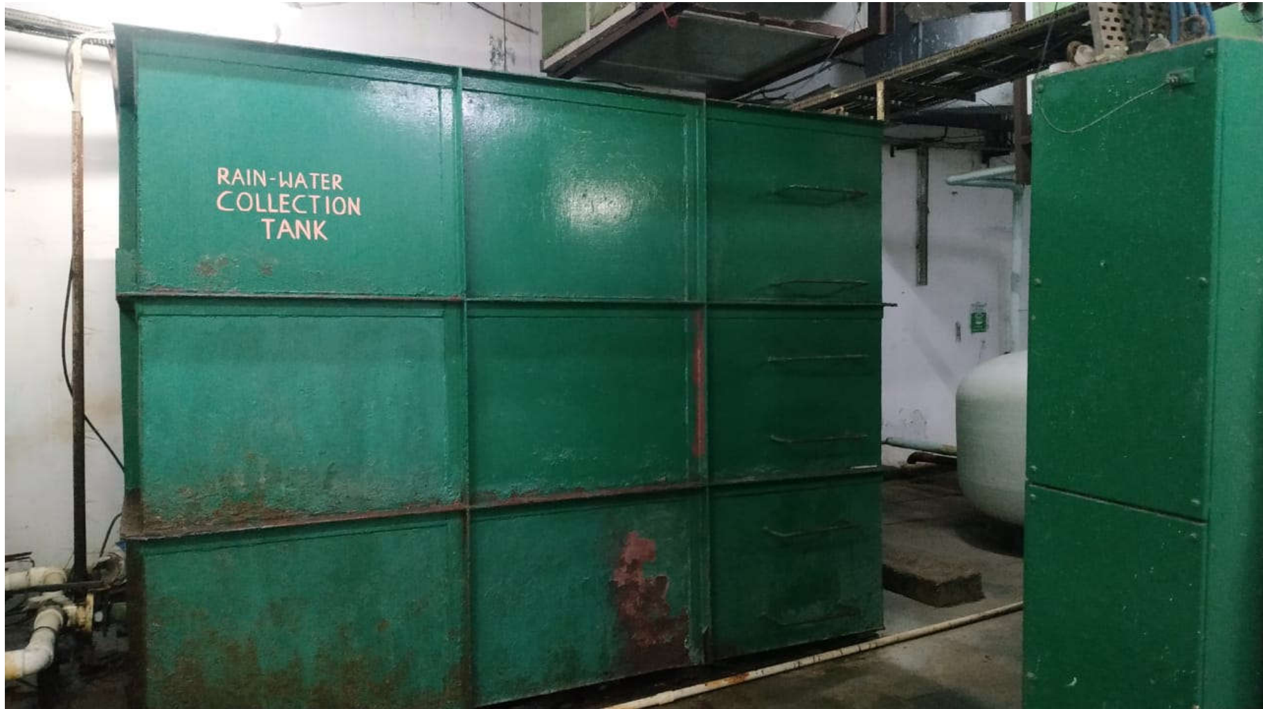
RAINWATER HARVESTING TANK PHOTOGRAPH
